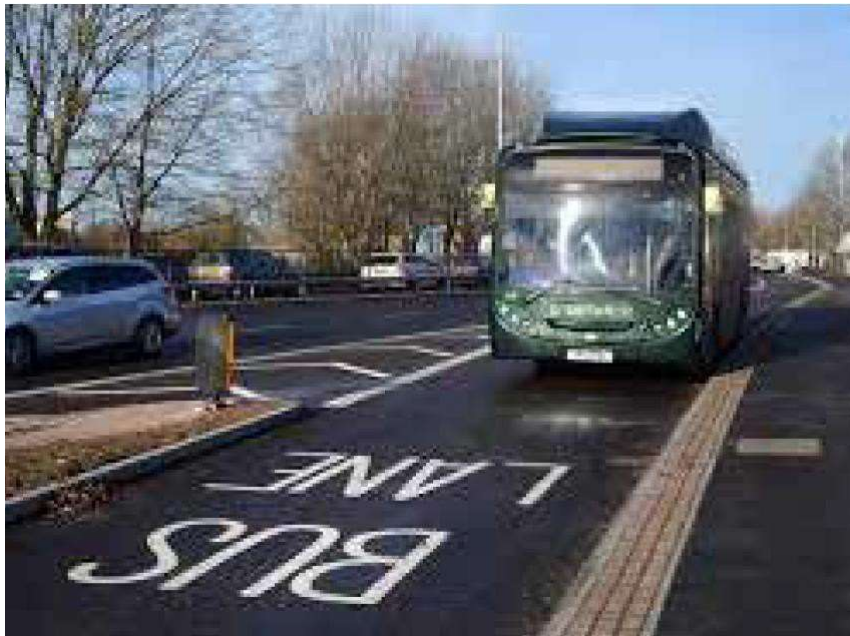
Figure 3-3: South Reading BRT bus lane
